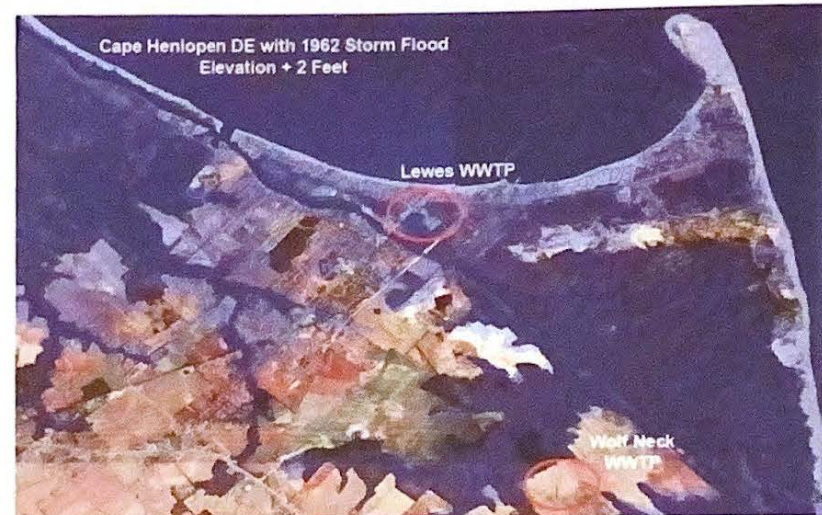
Fig. 1.23. Wastewater treatment plants in the area of Cape Henlopen DE are vulnerable to sea level rise. Using the 1962 storm flood elevation, this image shows that Lewes WWTP would be flooded and the facility at Wolf Neck would be nearly surrounded by water. Courtesy of David B. Carter, Coastal States Organization Climate Change Workgroup Co-Chair & Delaware Coastal Program Manager.
